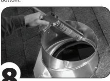
Seal the adjusting seam and the base/elbow connection seam on inside with roofing cement. Seal locking clamp holes and all exposed nails with roofing cement.
