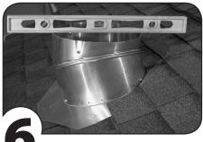
Rotate top of elbow to level position
