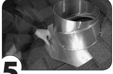
Slide top half of flashing under entire perimeter of hole with roofing cement. shingles. Secure with nails at top, sides and by turning counter clockwise. bottom.
