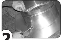
Align roof pitch number on elbow with the indicator line on the base flashing. Place 3 screws through holes that line up with predrilled holes in base.
