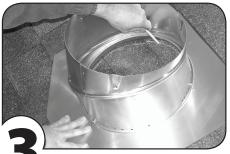
Locate base opening between rafters and mark hole to be cut. Locate rafters by tapping roof.
