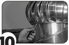
After installing, check to see that Whirlybird® turbine vent turns freely. In transportation it may have shifted slightly. If necessary, minor adjustment may be made by gently prying lowest point of turbine upward to remove any wobble.
